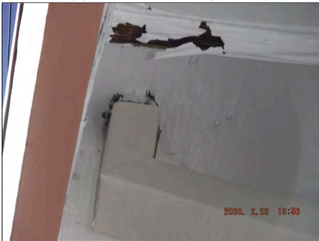
1.5(1) FASCIA / SOFFITS (Picture 3)
