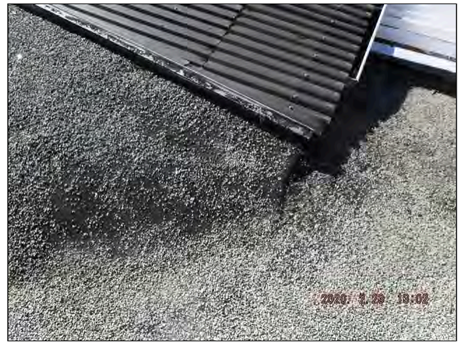
1.0 ROOF COVERING (Picture 2)
