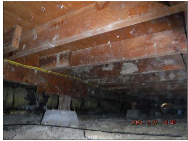
9.2 FLOOR FRAMING (Picture 1)
