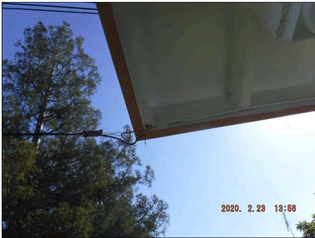
1.5(1) FASCIA / SOFFITS (Picture 1)
