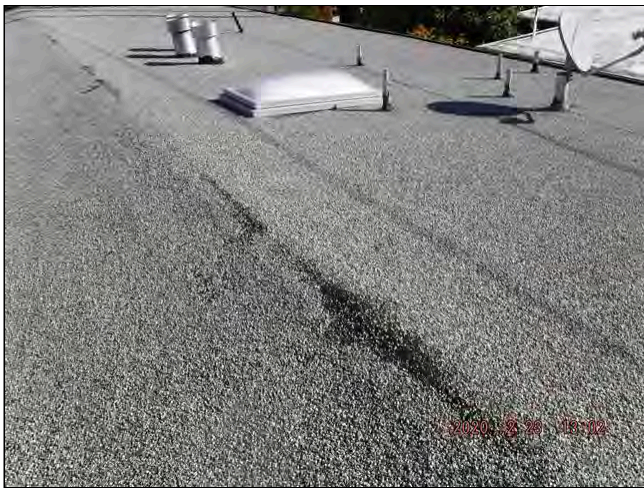
1.0 ROOF COVERING (Picture 1)
