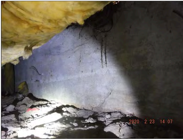
9.0 FOUNDATION WALLS (Picture 1)
