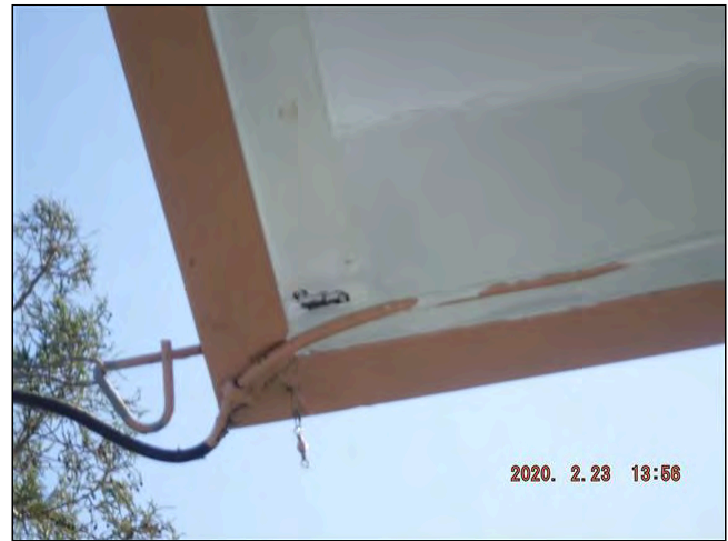
1.5(1) FASCIA / SOFFITS (Picture 2)
