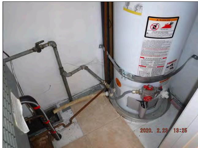
14.3 GAS / FUEL LINES AT UNIT (Picture 1)
