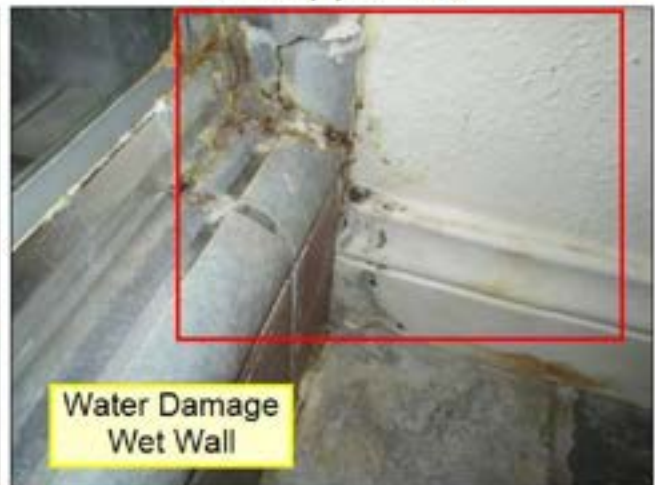
6.5 WALLS / CEILING Picture 1
