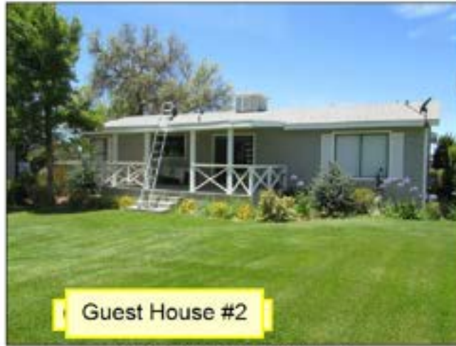
1.0.C ROOFING Picture 1
