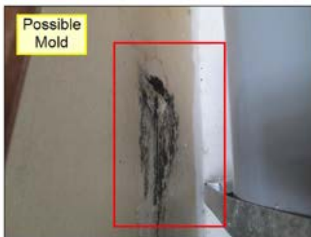
4.2.C WALLS / CEILINGS Picture 1
