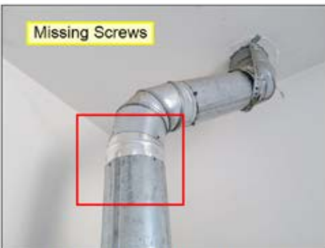
13.1.A VENT CONNECTOR Picture 1
