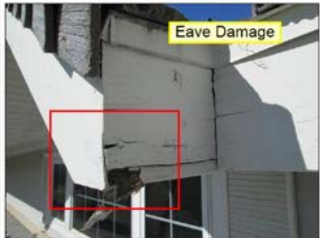
1.6.A FASCIA / SOFFITS Picture 1
