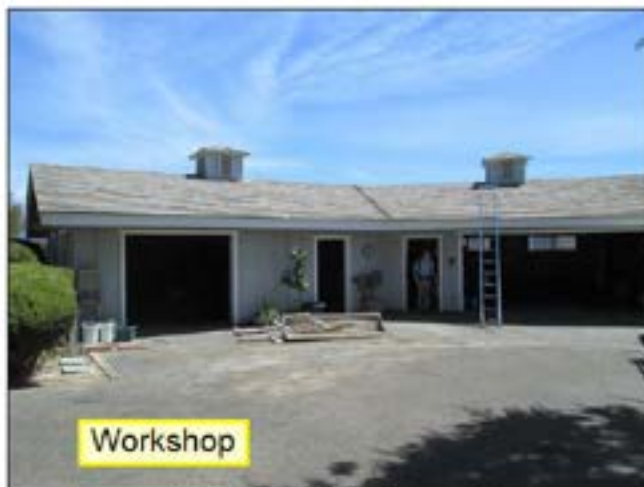
4.0.B ROOFING Picture 1
