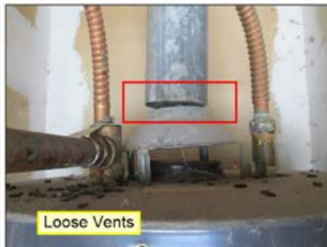
13.1.D VENT CONNECTOR Picture 1
