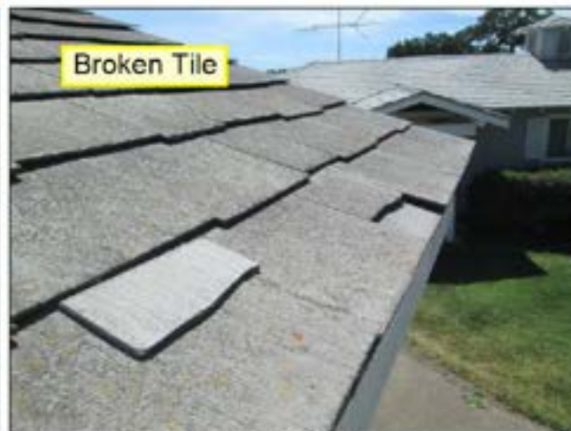
4.0.B ROOFING Picture 2
