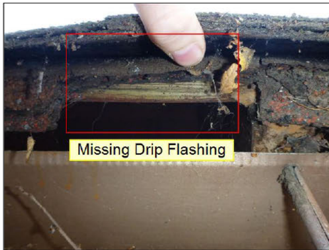
1.1 EXPOSED FLASHING (See Picture(s))
