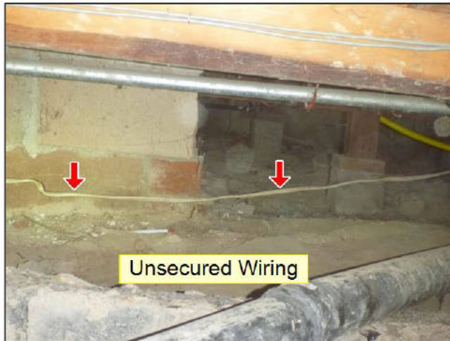
9.5 WIRING / CONDUCTORS (See Picture(s))
