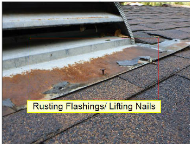
1.1 EXPOSED FLASHING (See Picture(s))
