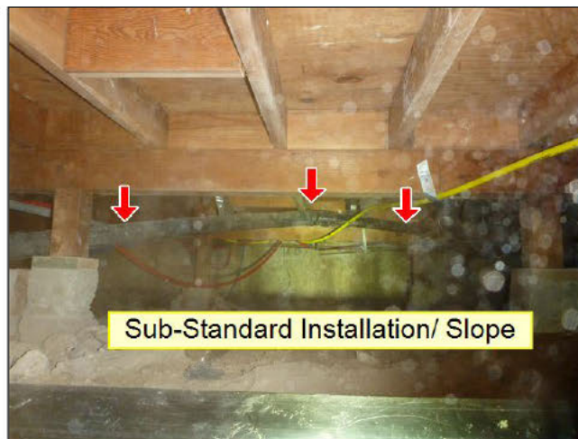
11.2 DRAIN / WASTE PIPING (See Picture(s))
