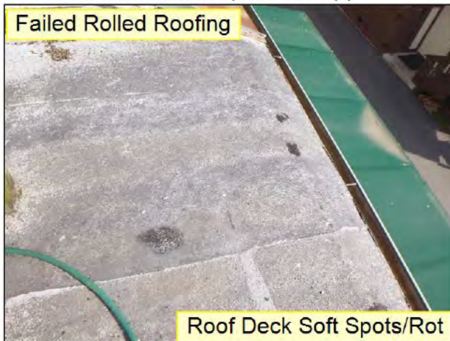
Failed Roofing
