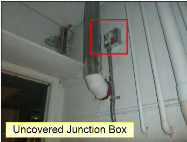
6.5 WIRING / CONDUCTORS (See Picture(s))
