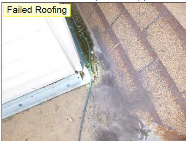
Roof Deck Soft Spots/Rot
