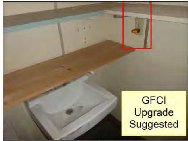
4.3 ELECTRIC / GFCI (See Picture(s))
