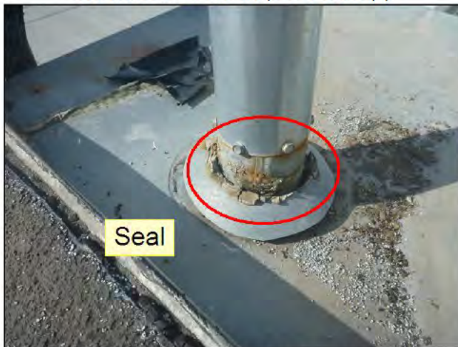
9.1 VENT CONNECTOR (See Picture(s))
