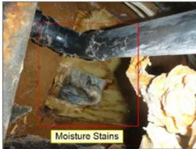
7.2 FLOOR FRAMING (See Picture(s))
