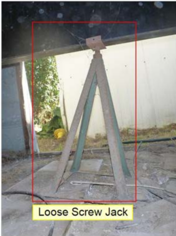
7.1 PIERS / COLUMNS (See Picture(s))
