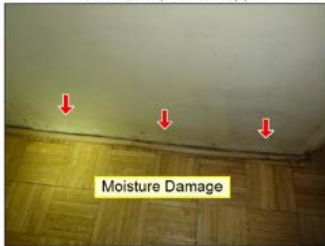
6.0 WALLS (See Picture(s))
