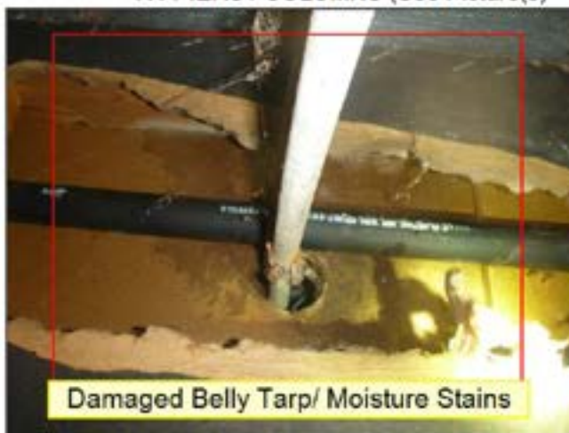
7.2 FLOOR FRAMING (See Picture(s))
