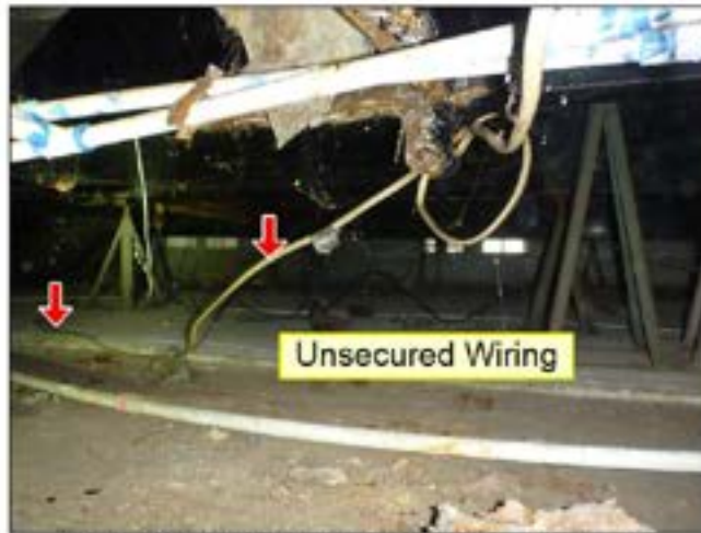
8.3 WIRING / CONDUCTORS (See Picture(s))
