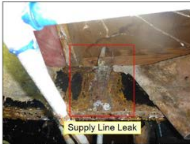
10.0 WATER PIPING (See Picture(s))
