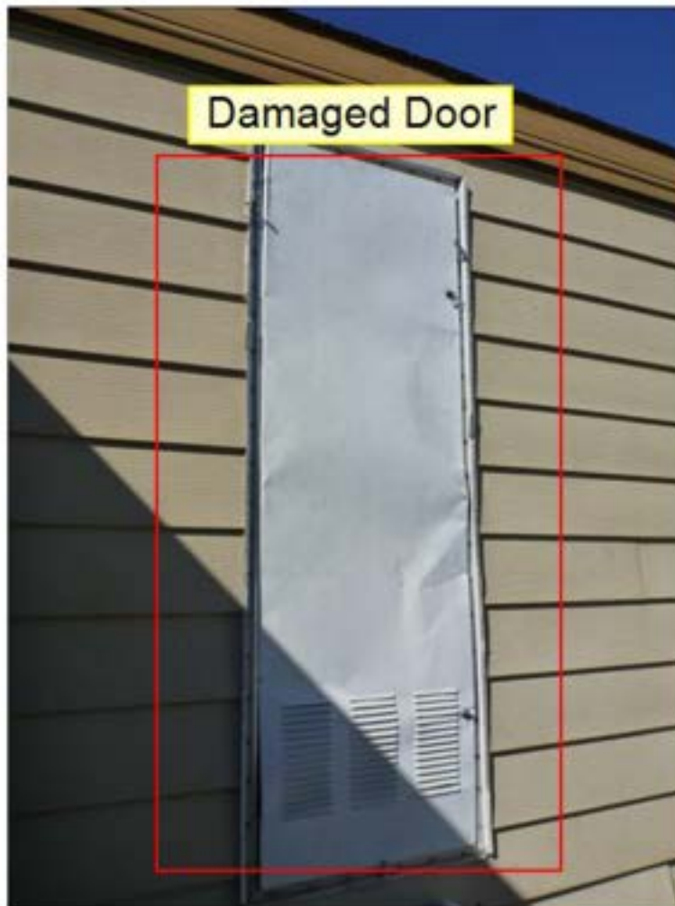
2.1 ENTRY DOORS (See Picture(s))
