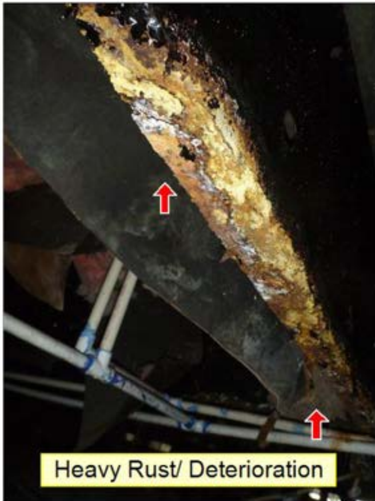
7.0 FOUNDATION (See Picture(s))
