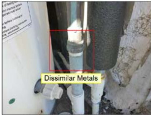
10.0 WATER PIPING (See Picture(s))
