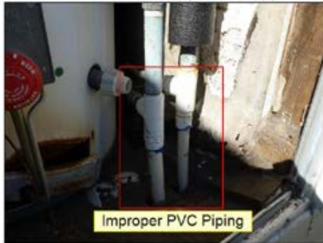
10.0 WATER PIPING (See Picture(s))
