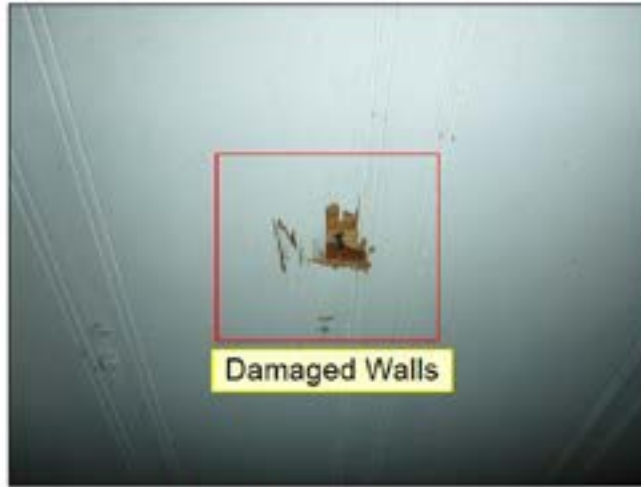
6.0 WALLS (See Picture(s))
