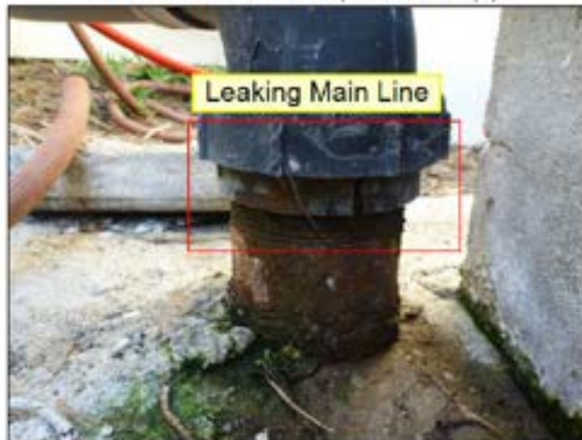
10.1 DRAIN / WASTE PIPING (See Picture(s))
