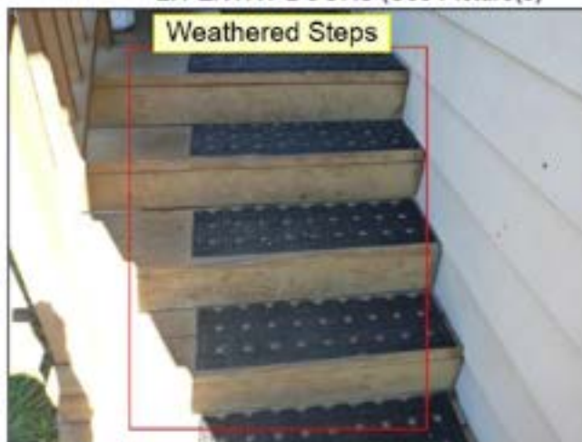
2.2 STAIRS / STOOPS (See Picture(s))
