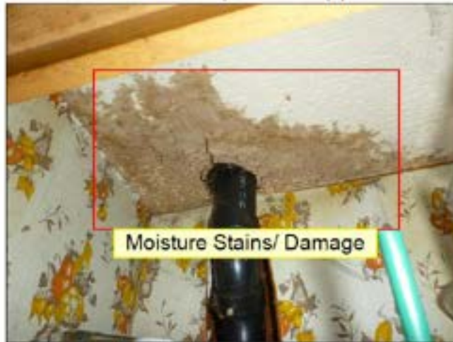
6.1 CEILINGS (See Picture(s))
