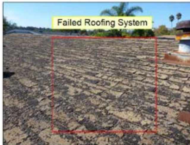
1.0 ROOFING (See Picture(s))
