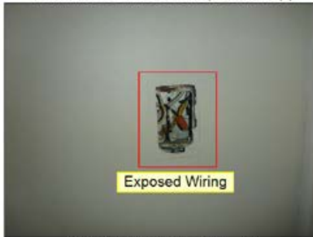
6.4 SUBPANEL(S) (See Picture(s))
