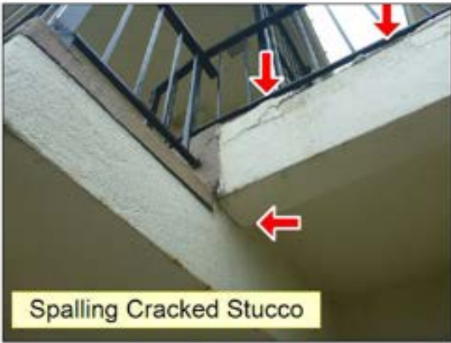
Damaged Stucco/Exposed Roof Sheathing
