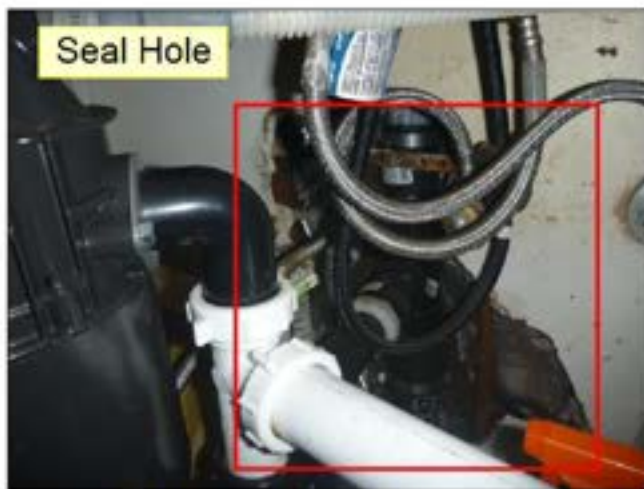
4.1.V WALLS / CEILING (See Picture(s))
