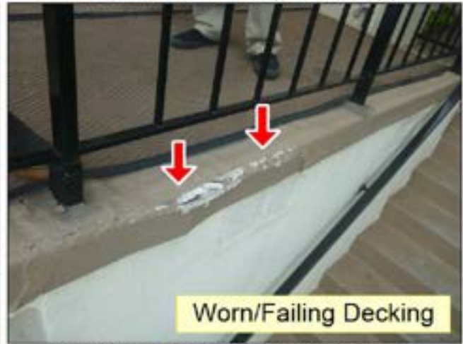
1.3 PORCH(ES) / DECK(S) (See Picture(s))
