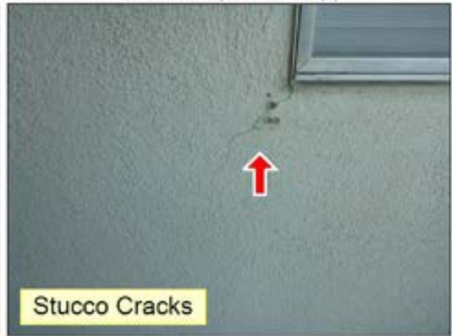
Damaged Stucco
