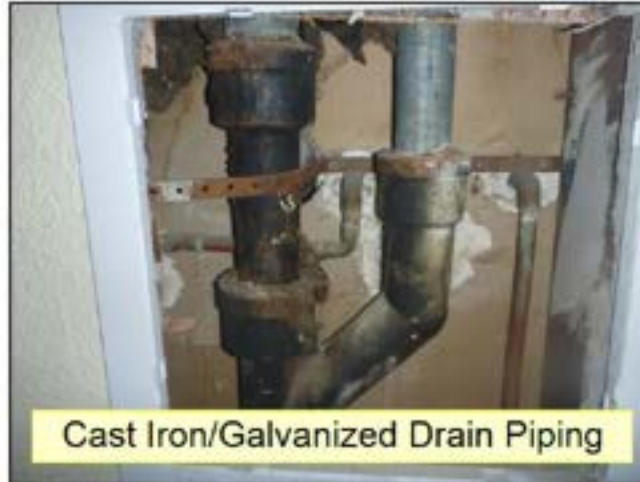
Original Cast Iron Drain Piping
