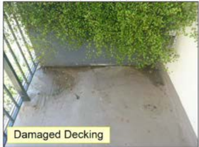
1.3 PORCH(ES) / DECK(S) (See Picture(s))
