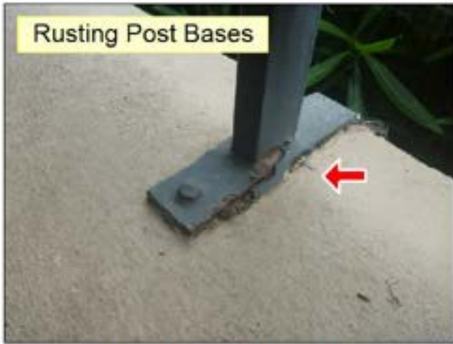
1.4 RAILINGS (See Picture(s))
