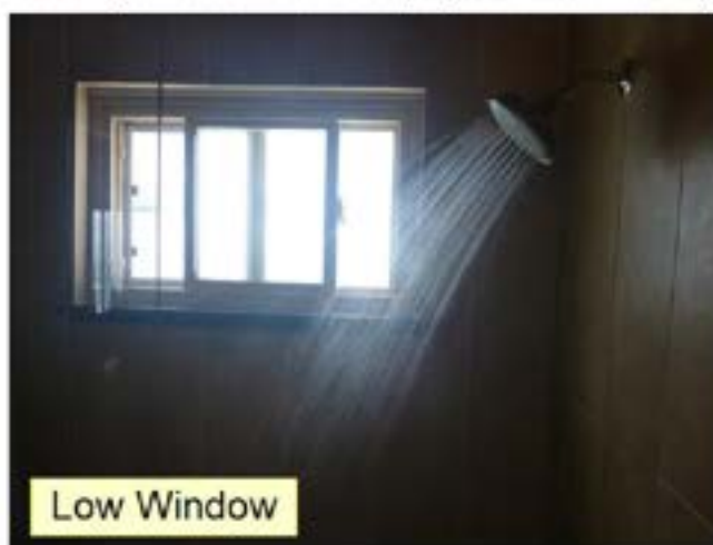
3.5.B VENTILATION (See Picture(s))
