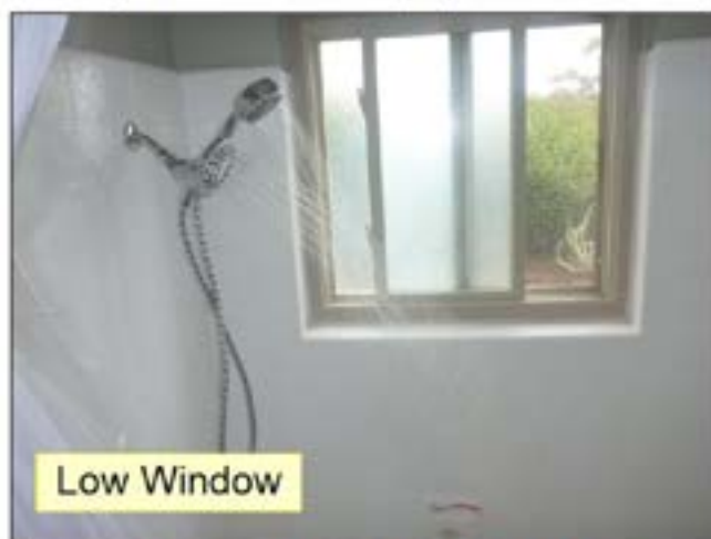
3.4.E VENTILATION (See Picture(s))
