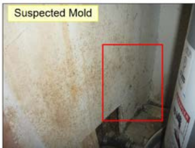
9.0.M WATER HEATER (See Picture(s))
