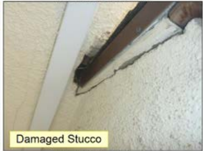
Damaged Stucco/Exposed Roof Sheathing
