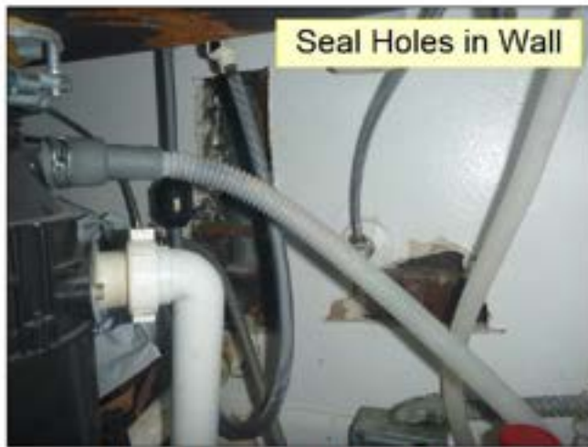
4.1.M WALLS / CEILING (See Picture(s))
