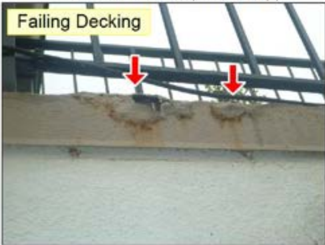
1.3 PORCH(ES) / DECK(S) (See Picture(s))
