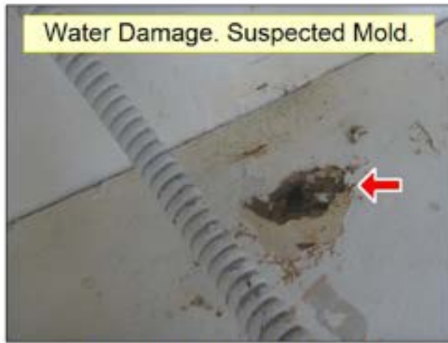
4.0.BB PLUMBING / SINK (See Picture(s))
