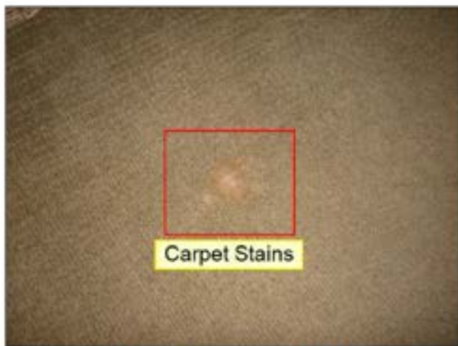
5.2 FLOORS (See Picture(s))
