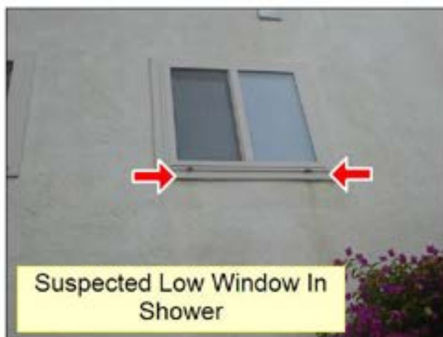
3.5.I VENTILATION (See Picture(s))
