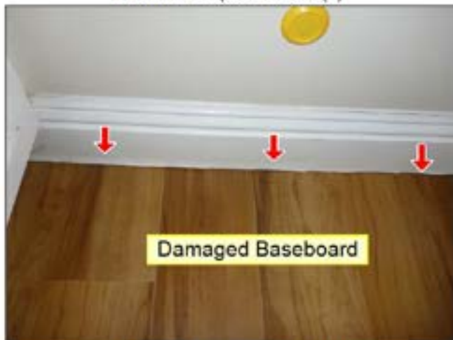
5.0 WALLS (See Picture(s))
