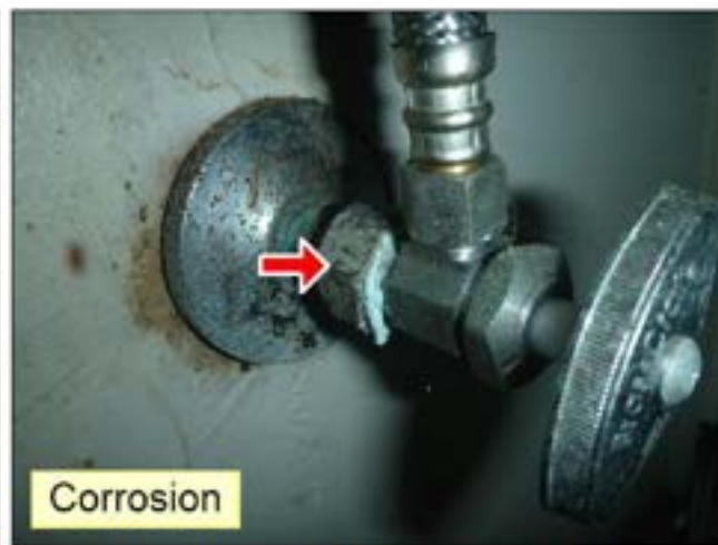
4.1.V WALLS / CEILING (See Picture(s))
