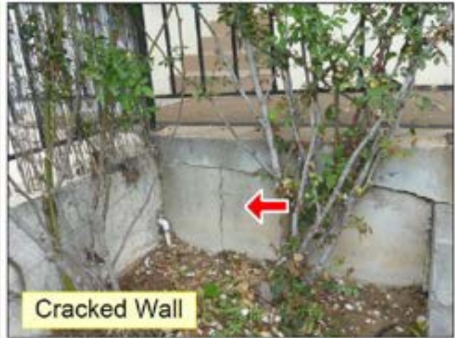
2.2 RETAINING WALL(S) (See Picture(s))
