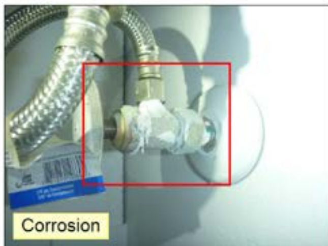
4.0.E PLUMBING / SINK (See Picture(s))
