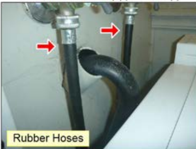
8.5 LAUNDRY (See Picture(s))
