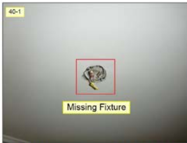
6.3 WIRING / CONDUCTORS (See Picture(s))
