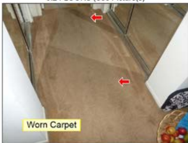
5.2 FLOORS (See Picture(s))
