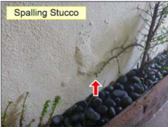
2.2 RETAINING WALL(S) (See Picture(s))
