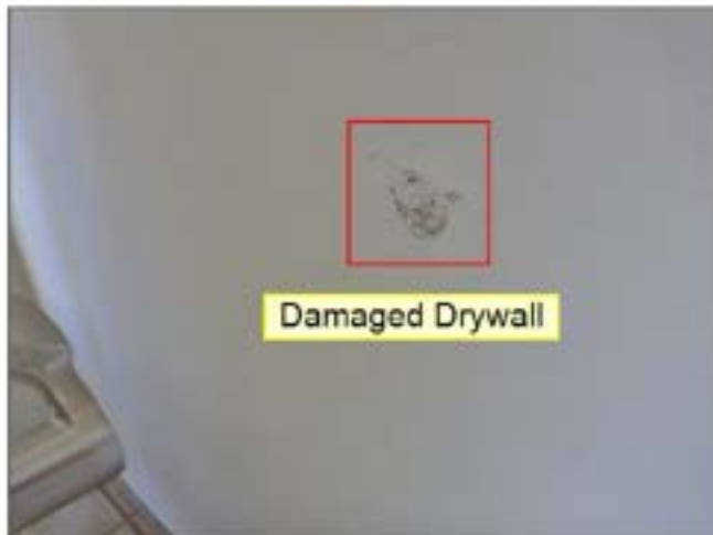
5.0 WALLS (See Picture(s))
