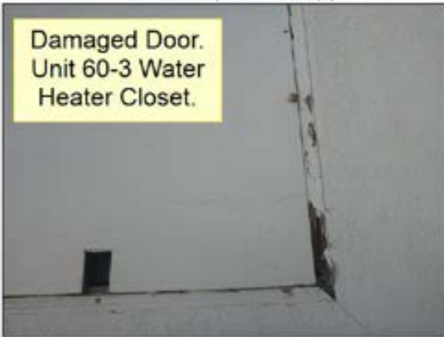
Water Staining. Mold.
