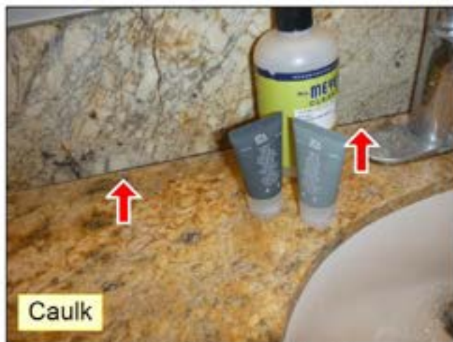
3.0.J SINK(S) (See Picture(s))
