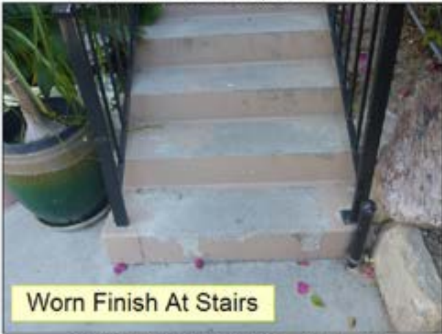
1.2 STAIRS / STOOPS (See Picture(s))
