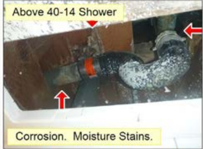
8.3 DRAIN / WASTE PIPING (See Picture(s))
