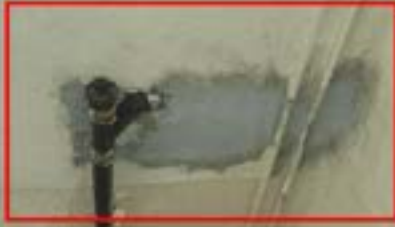
Plumbing Repair. Building 60.
