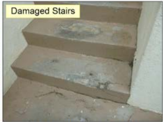
1.2 STAIRS / STOOPS (See Picture(s))
