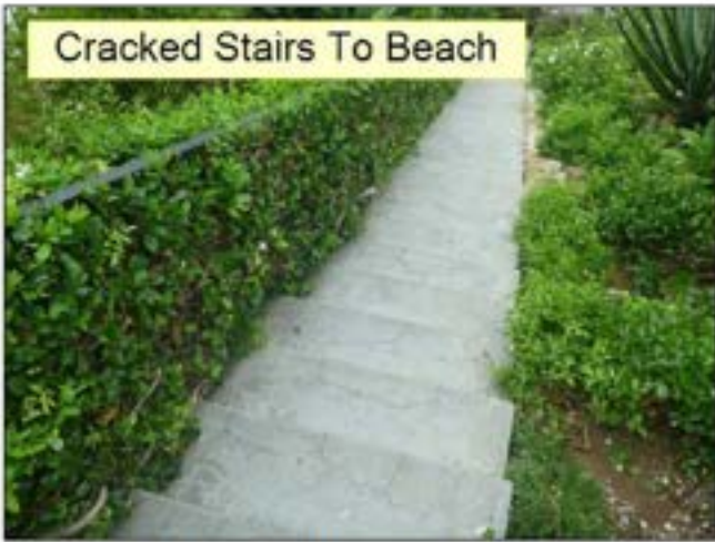
1.2 STAIRS / STOOPS (See Picture(s))
