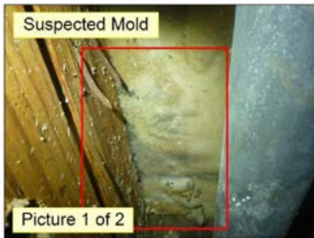
3.4.D WALLS / CEILING (See Picture(s))
