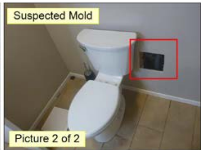
3.4.D WALLS / CEILING (See Picture(s))
