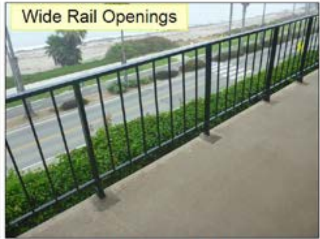
1.4 RAILINGS (See Picture(s))
