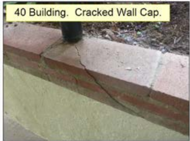
2.2 RETAINING WALL(S) (See Picture(s))
