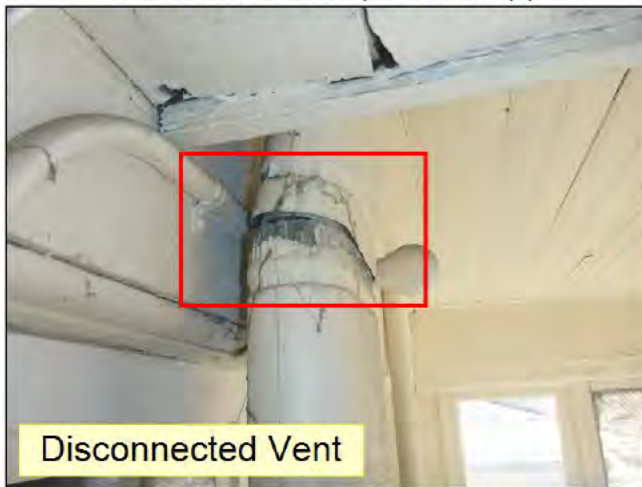
6.2 VENT CONNECTOR (See Picture(s))
