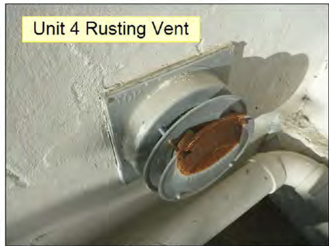
6.2 VENT CONNECTOR (See Picture(s))
