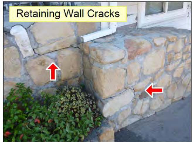
3.4 RETAINING WALL(S) (See Picture(s))
