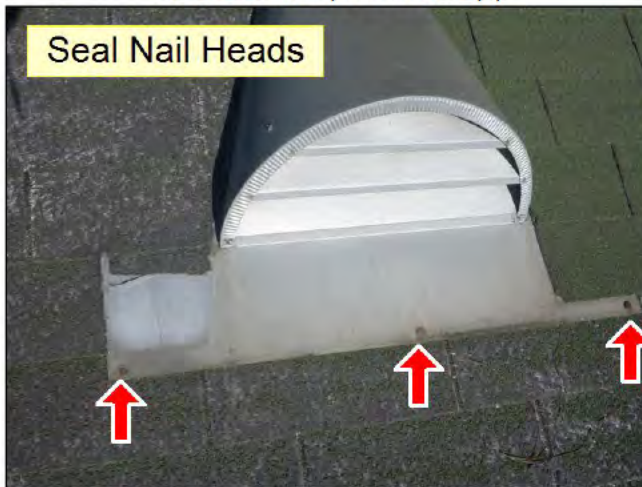
1.1 EXPOSED FLASHING (See Picture(s))
