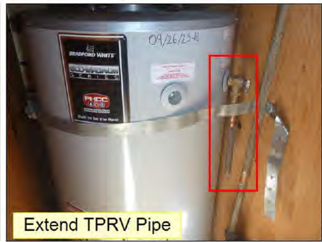
4.3 SAFETY VALVE PROVISIONS (See Picture(s))
