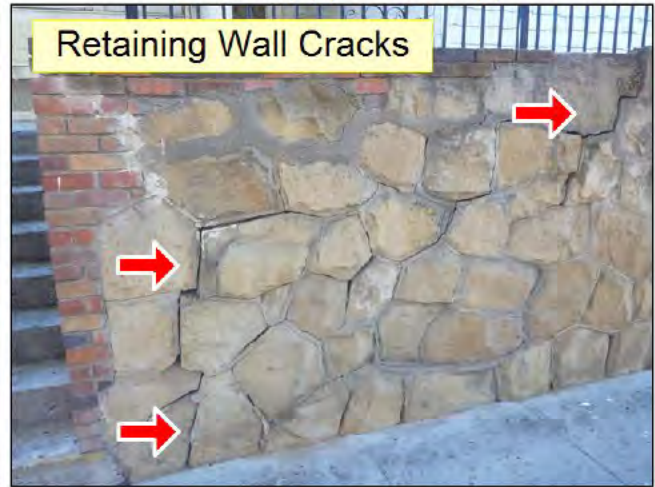
3.4 RETAINING WALL(S) (See Picture(s))
