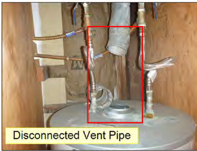
4.1 VENT CONNECTOR (See Picture(s))
