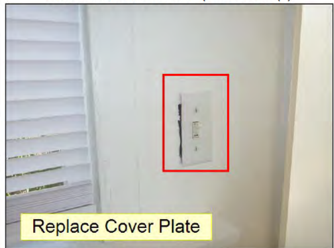
8.6.D ELECTRIC / GFCI (See Picture(s))
